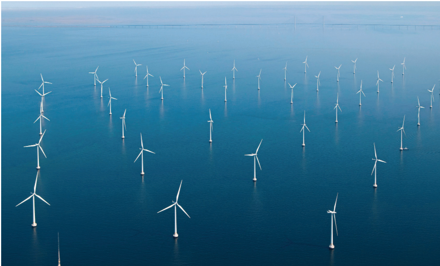
(Left: Lillgrund Wind Farm, 10 km off the coast of southern Sweden below the Öresund Bridge, which connects Copenhagen to Malmö. It has 48 wind turbines and a total capacity of 110 MW (megawatts). They are 115m tall, and can meet the capacity of 60,000 homes.)
